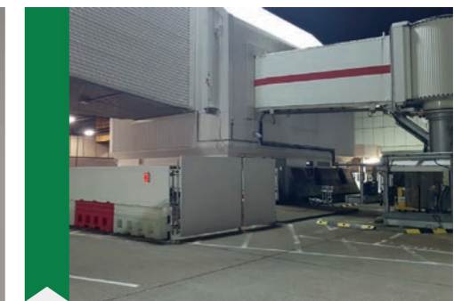
Project - Airside storage facility Hoarding Systems - Plasblok
