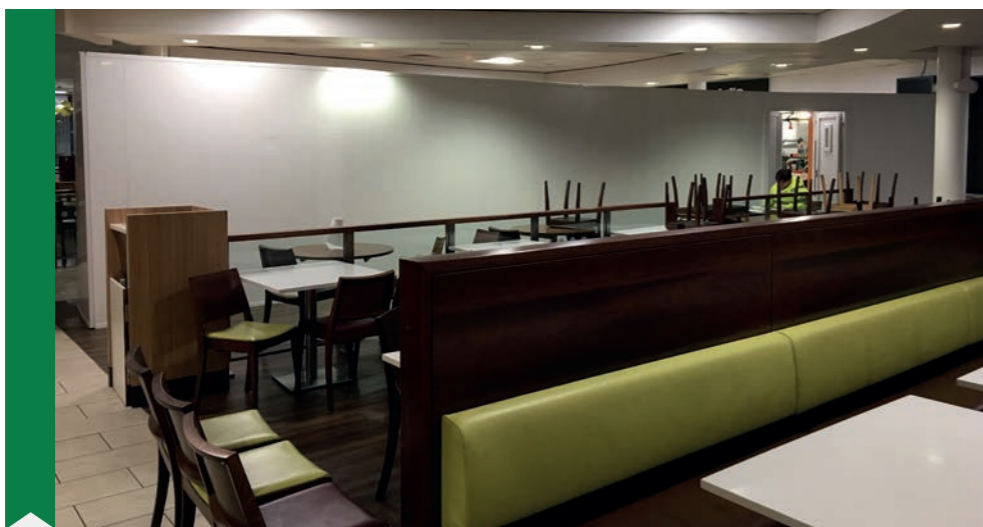
Project - McDonalds refit Hoarding Systems - Internal
