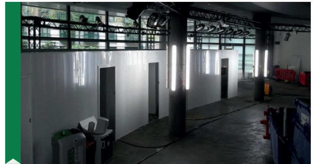
Project - Café refit Hoarding Systems - Internal
