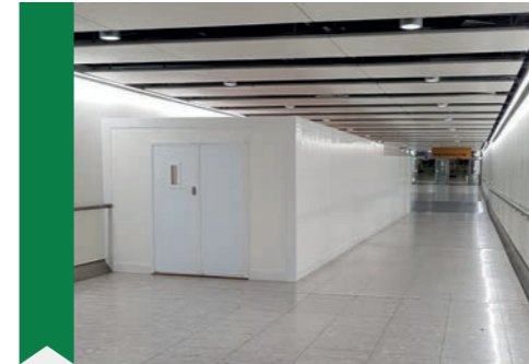
Project - LUL Hoarding Systems - Scaffold based internal
