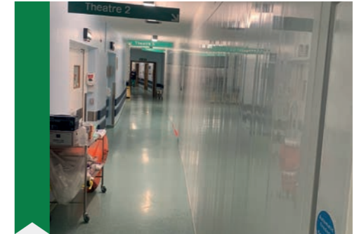
Project - Lab refurbishment Hoarding Systems - Internal
