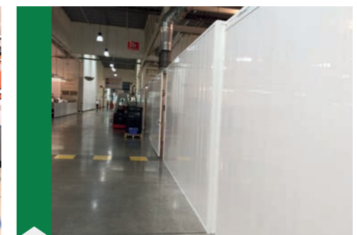
Project - Manufacturing line segregation Hoarding Systems - Bespoke internal system / Sliding door
