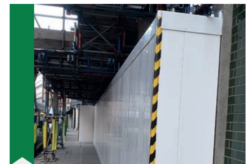
Project - Office refurbishment #Hoarding Systems - Plasklad
