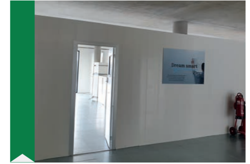
Project - Office refurb, Site set up Hoarding Systems - Internal
