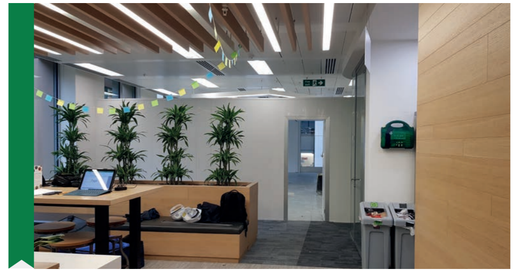
Project - Office refurbishment, Site set up Hoarding Systems - Internal
