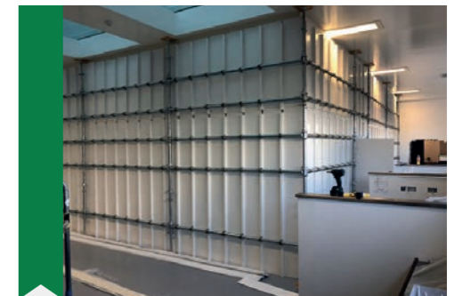
Project - Central decontamination unit Hoarding Systems - Demo wall
