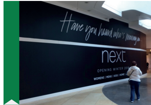
Project - Store demolition Hoarding Systems - Demo wall
