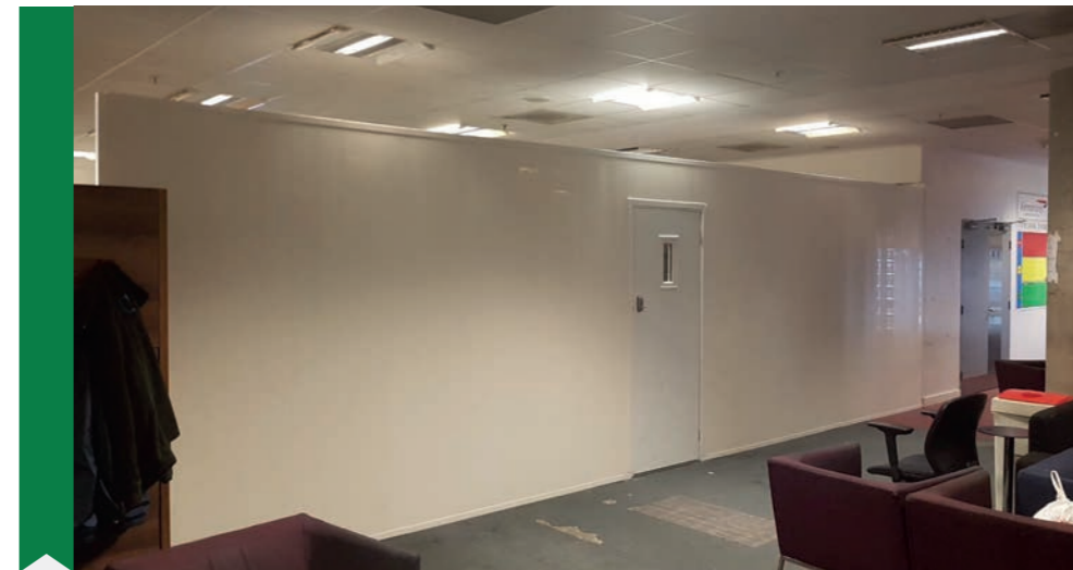
Project - BAA Staff lounge Hoarding Systems - Internal
