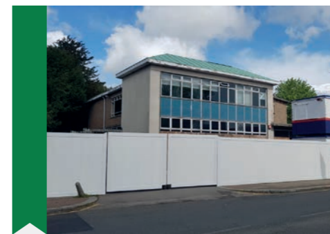
Project - Building demolition Hoarding Systems - External
