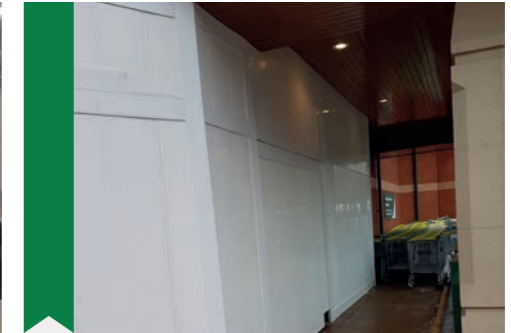
Project - WMS Extension Hoarding Systems - Demo wall
