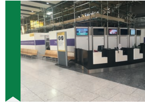
Project - Ceiling replacement Hoarding Systems - Internal
