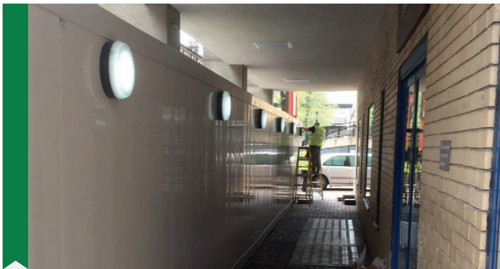
Project - Royal Birth of Prince George, Paparazzi screening Hoarding Systems - Internal
