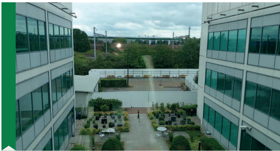
Project - Office refurbishment Hoarding Systems - External
