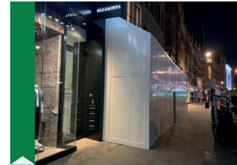
Project - Store refit Hoarding Systems - Demowall/ Roof
