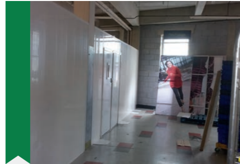
Project - Store refresh Hoarding Systems - Internal
