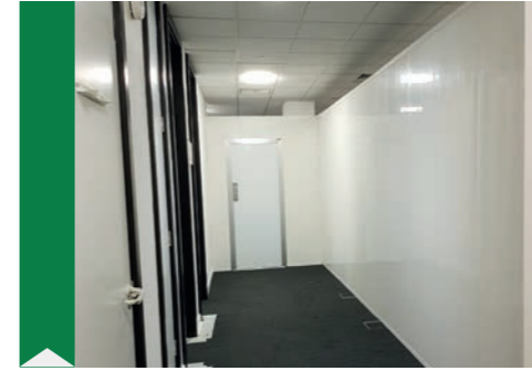
Project - Office refurb, Site set up Hoarding Systems - Internal
