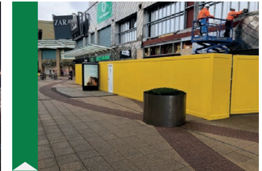
Project - Exterior cladding Hoarding Systems - External
