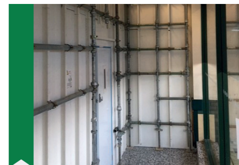
Project - WMS Extension Hoarding Systems - Demo wall
