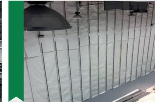
Project - Dyson R&D extension Hoarding Systems - Demowall – Firefly
