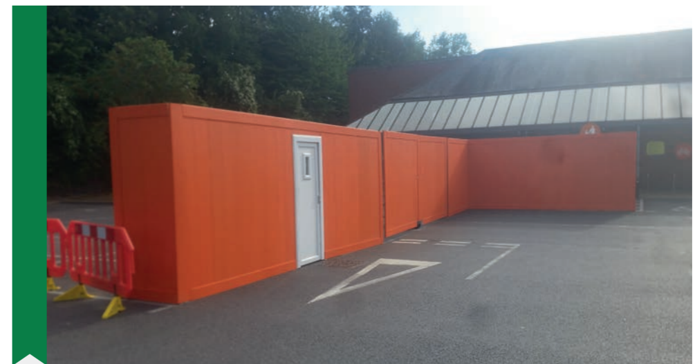
Project - SSL Extension Hoarding Systems - External
