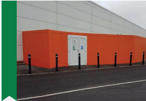
Project - Store refresh Hoarding Systems - External
