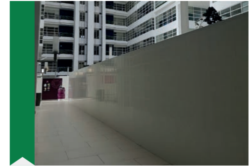
Project - Flooring replacement Hoarding Systems - Internal
