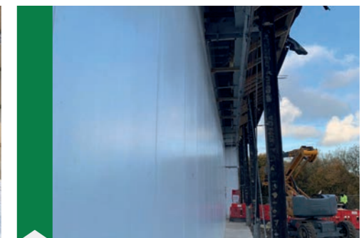
Project - WMS Extension Hoarding Systems - 1hr Fire rated composite
