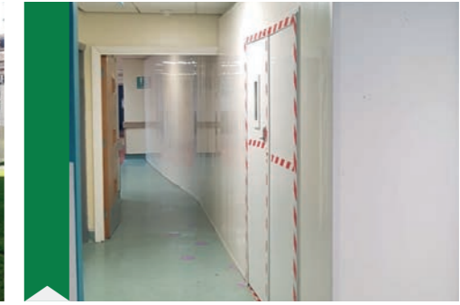
Project - A&E Hoarding Systems - Internal
