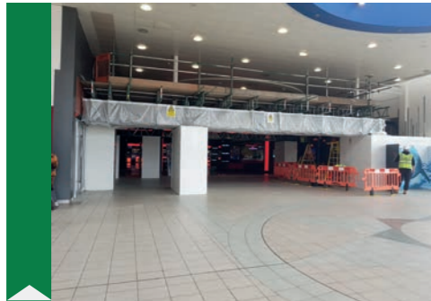
Project - Ceiling works Hoarding Systems - Plasklad
